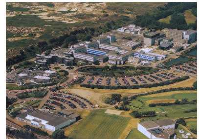
ESA technology centre (ESTEC), Noordwijk
